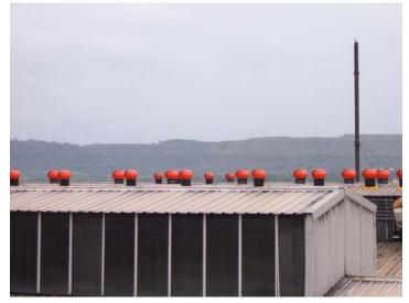
**Result**: The 24 Nos. \* SVS-14 Wind Driven Turbo Ventilators achieved the objective set. Client placed repeat order for 48 Nos. within a fortnight of initial order installation. Client has further increased the quantity by 24 numbers to bring the total quantities installed to 96 nos. Client has reported reduction in temperature & smoke / fume levels and better visibility.
